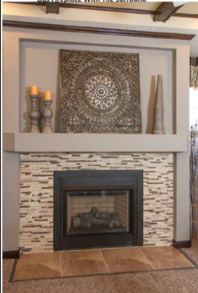
Gas Fireplace With Tile Surround
